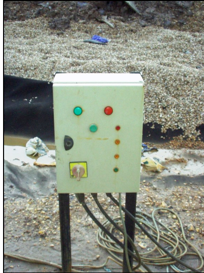
Photo 19: Control panel showing signs of corrosion
