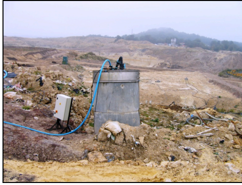
Photo 16: Control panel installed too close to leachate chamber
