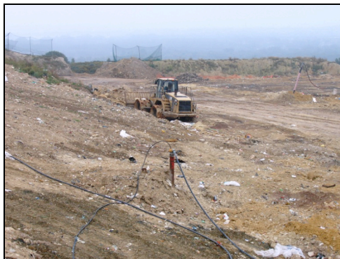
Photo 17: Unprotected leachate extraction point
