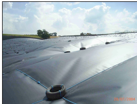
Photo 2: 'Ballooning' due to landfill gas collecting under geo-membrane
