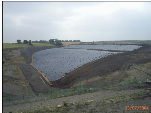
Photo 3: Completed capped cell
