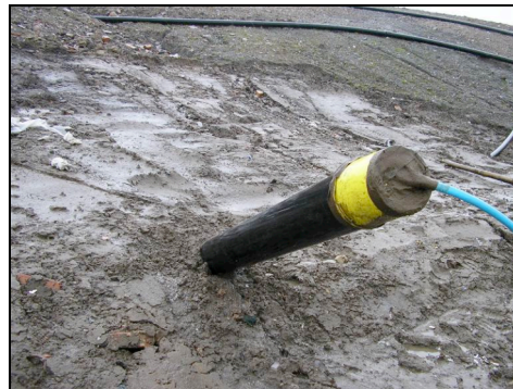
Photo 23: Poor Design - bucket used as a head works and sealed with tape
