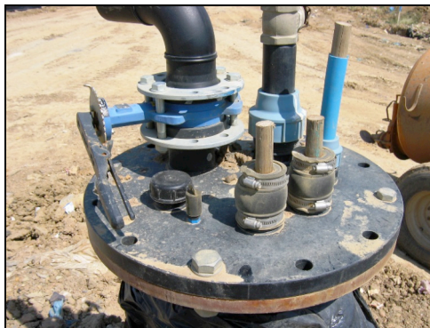
Photo 14: Poor standards of installation
